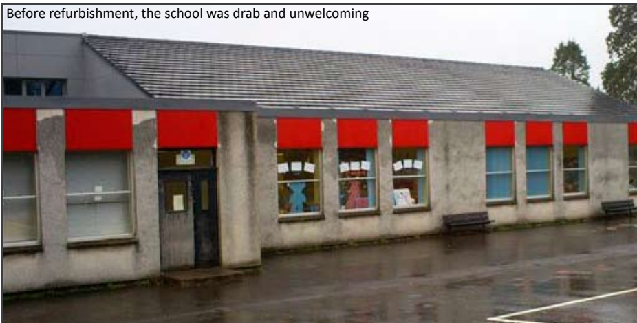
Before refurbishment, the school was drab and unwelcoming
